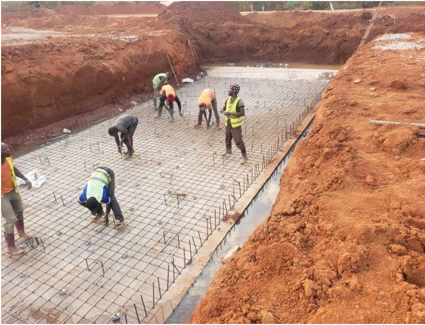
Preparation of bottom slab reinforcement after casting a blinding concrete in box culvert
