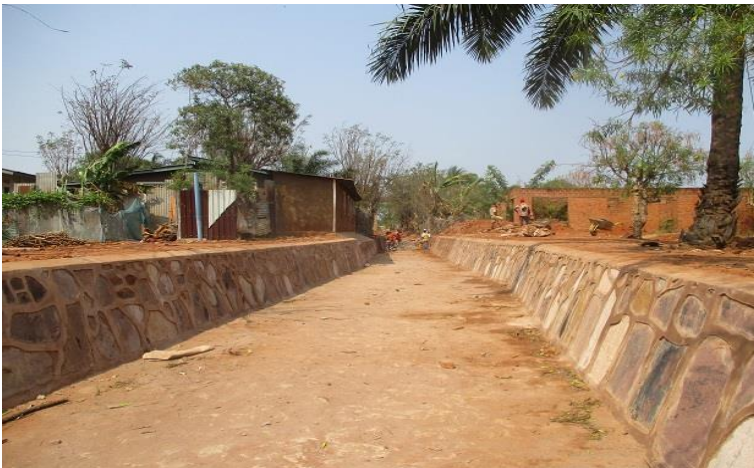
Repaired Grouted Stone Pitching
