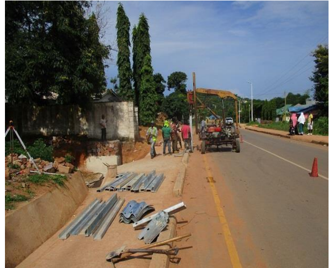
Fixing of Guardrail
