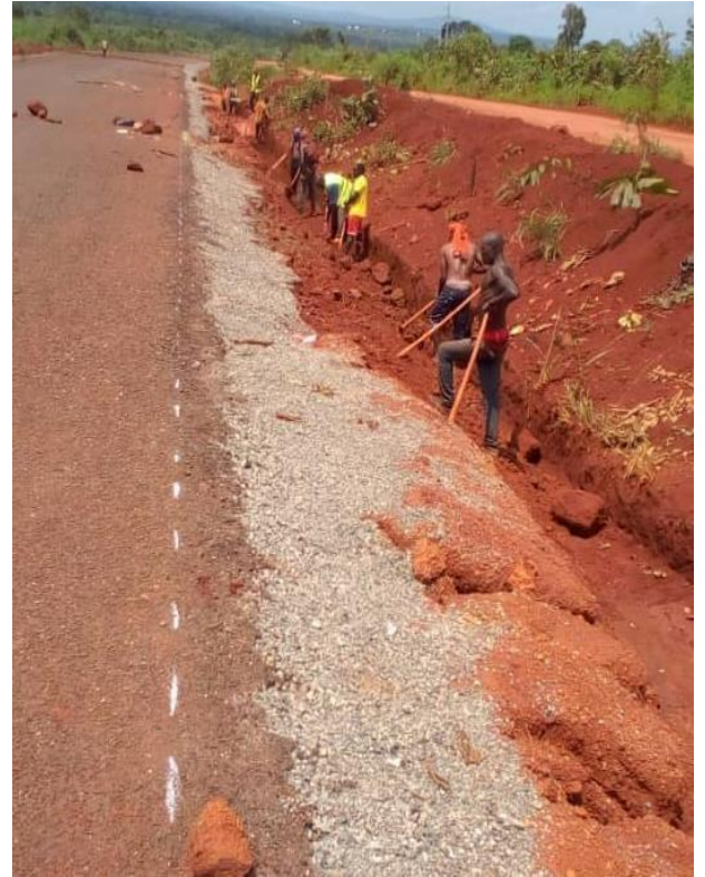
Trimming of excavations for concrete side drains
