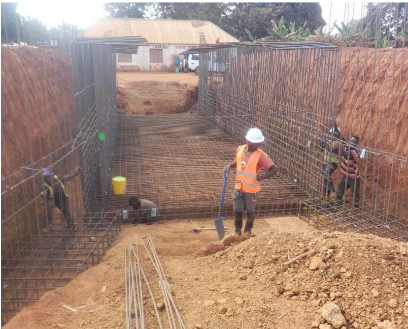
Fixing Reinforcement for the Underpass
