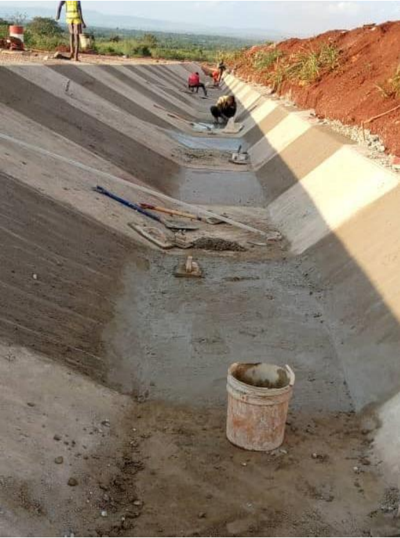
Cast and Class U2 surface finish for concrete side drain
