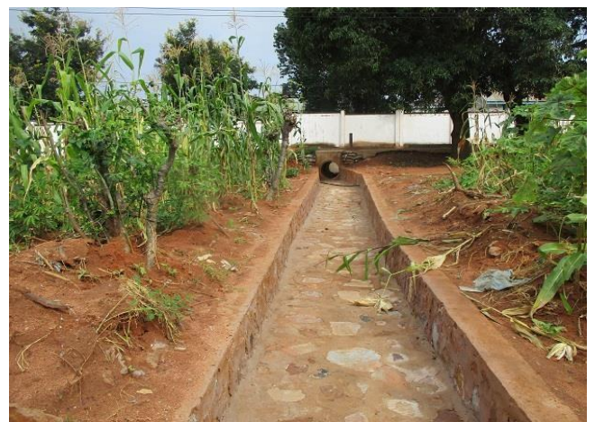
Extension of Pipe culvert outfall
