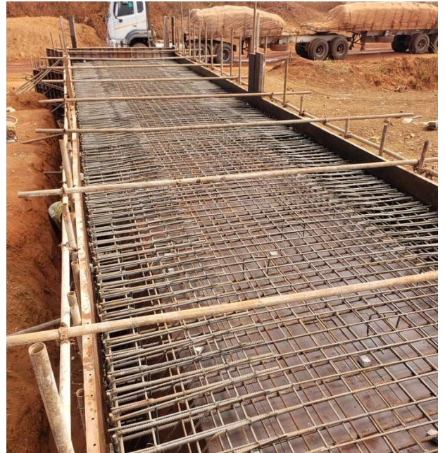
The casting of concrete in the process after fixing reinforcement and formwork for vertical walls and top slab
