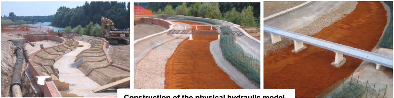
Construction of the physical hydraulic model
